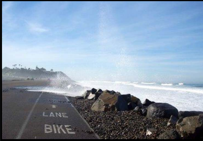
Current overtopping and flooding of HWY 101 at the Project site
