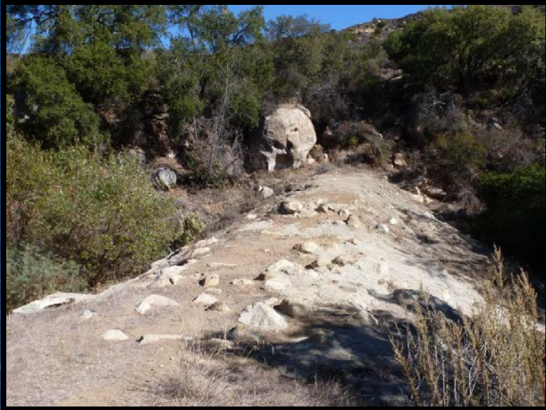
Rattlesnake Creek Debris Basin: Grouted Rock Dam
